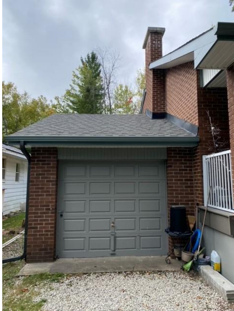
Site Photo 1 – Existing Attached Garage
